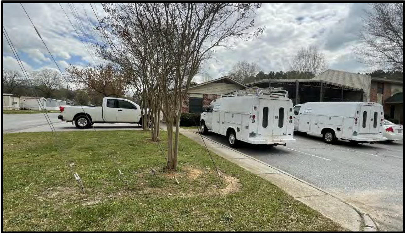
Photo 4—the maintenance building
