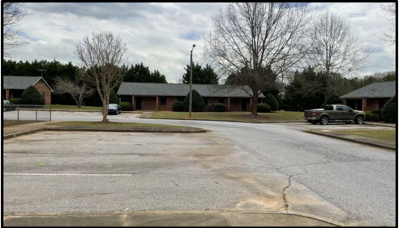
Photo 9—the site from the community center
