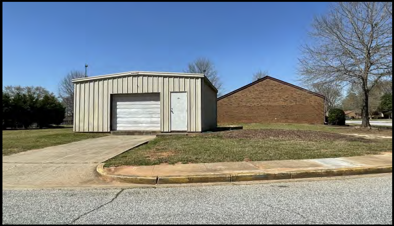
Photo 9—the maintenance building
