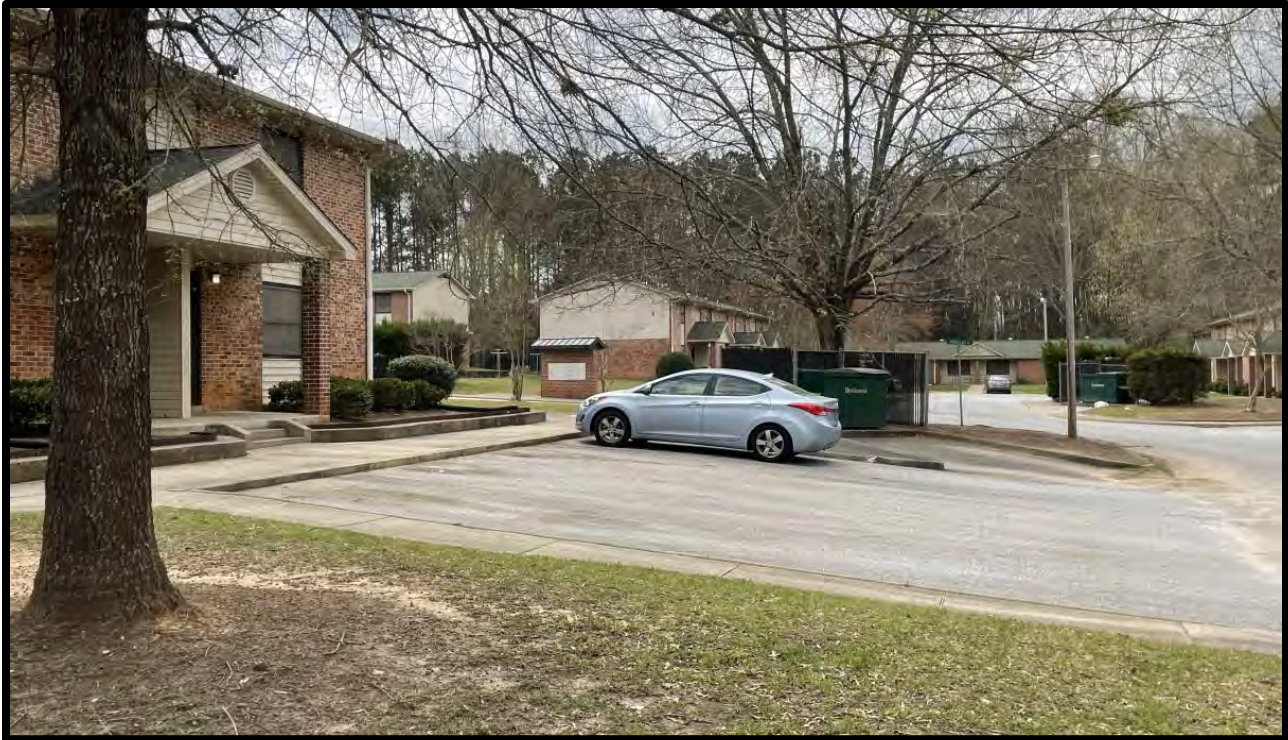
Photo 3—two-story buildings on the site
