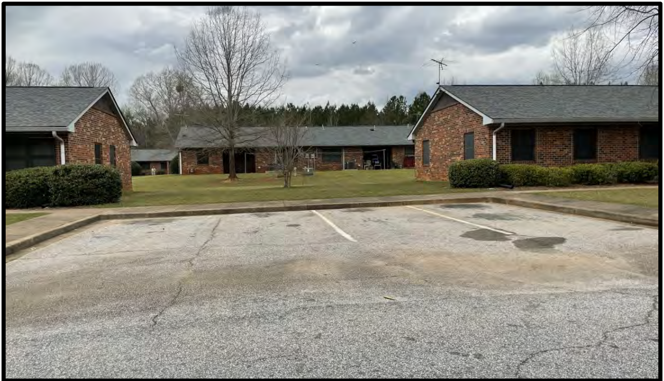
Photo 8—the site from Burgess Drive
